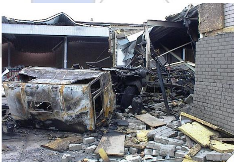
Fig. 1: Linde N 2 O Tanker Explosion
