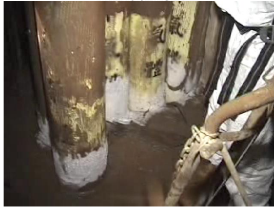
Fig 8: Removing ammonia cylinders frozen to ground
