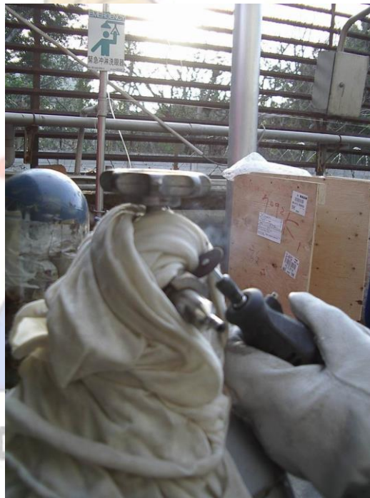
Photo of Dremel tool being used to cut a nut. (towels protecting valve are not necessary, but won't hurt)
