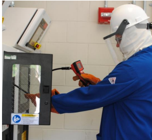
Fig. 22: Fiberoptic Scope Inspection
